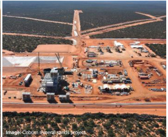
Image: Coburn mineral sands project.
